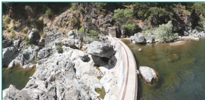
DeSabra–Centerville, located on Butte Creek in the northern Sacramento Valley has a complex system of dams, canals, reservoirs, and power generation facilities. These hydro-electric projects that have been operated by PG&E for over 100 years are now for sale. Photo by Allen Harthorn, Friends of Butte Creek
