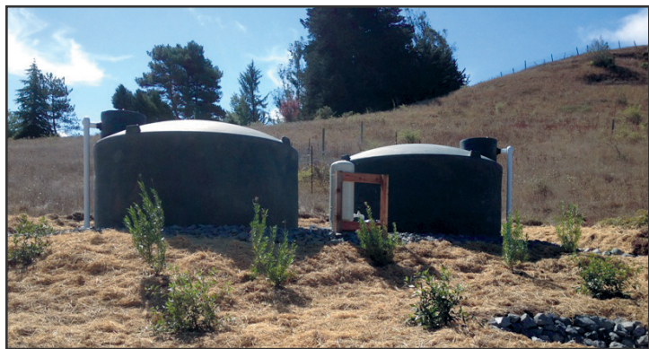
Rainwater catchment tanks to store winter water for summer use. Photo: John Green
