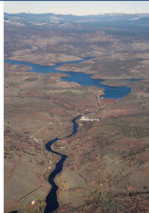
Iron Gate dam on the Klamath River Photo by Thomas B. Dunklin
