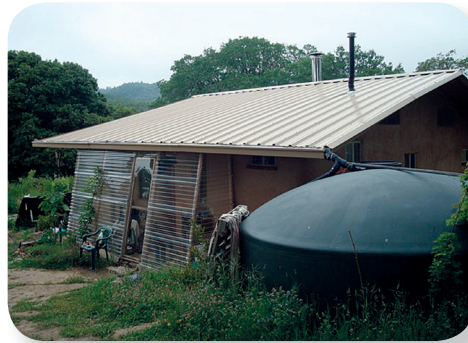
Roofwater rain catchment is a great way to capture and store water.
