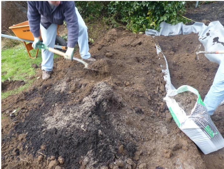
Figure 9. A few inches of compost and a sprinkling of a soil restoration product with mycorrhizae and biota (Permamatrix used here) were placed over native soils, then shoveled together and into the swale.
