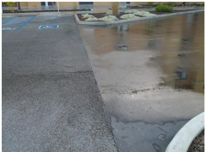
Figure 7: Pervious pavement (left side) and traditional impervious pavement (right side). Areas of pooled water are seen on the impervious surface.
