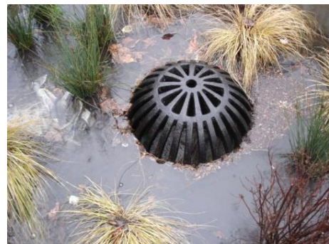
Figure 1 Avoid bark mulch. It floats, carrying pollutants adhered to its surface to downstream waterways.
