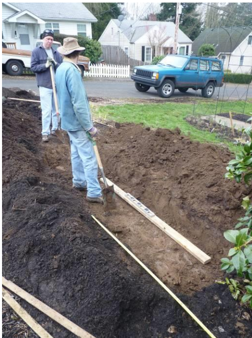
Figure 8. Since the bottom of the lined swale will empty into native soil, the bottom of the swale must also slope away from the building. Otherwise, plant roots won't dry out between waterings and rainfall events or plants won't be healthy.
