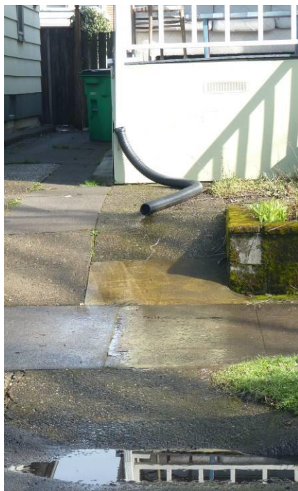
Figure 4 Avoid disconnecting your downspout to impervious areas. This has as little benefit to the watershed and could create safety hazards (e.g., puddle at the bottom of the driveway).
