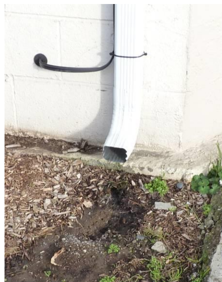
Figure 3 Placing a downspout this close to a slab is not ideal. It would require a vertical liner to be placed at least a few inches deeper than the slab section (including rock). If erosion like this occurs, spread the flows out and/or plant some vegetation at the mouth.
