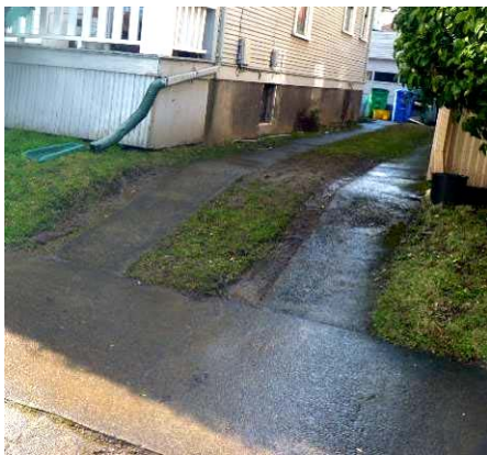
Figure 2. Lawn tends to get compacted when not properly designed and will not grow in the place where you most often park your car.
