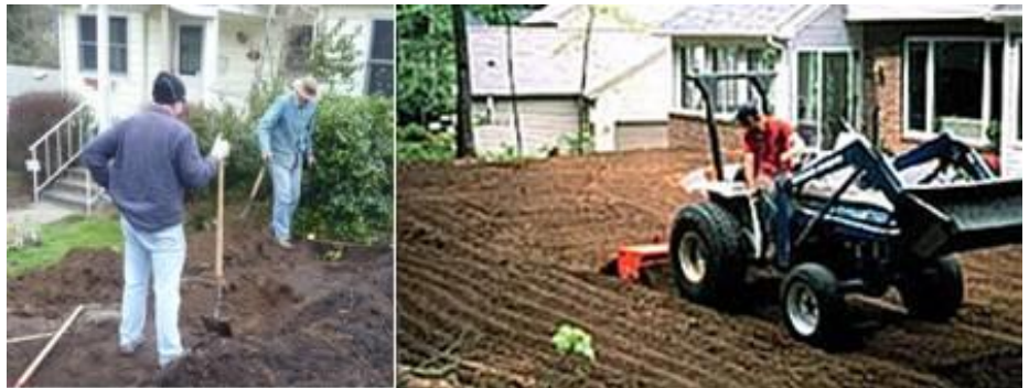
Figures 4 & 6. A range of construction equipment (tiller, cat mounted ripper, tractor-mounted disc, etc) or simply shovels and rakes may be used depending on the extent of the area to be amended.
