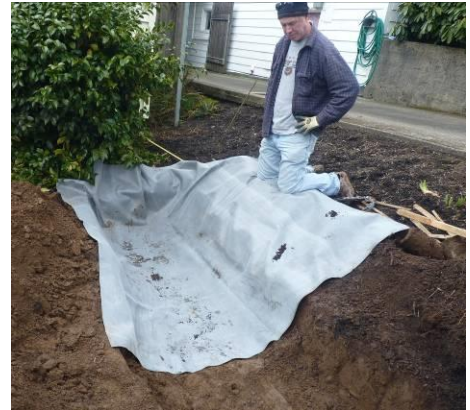
Figure 7. A single sheet of EPDM is being laid in the bottom to a minimum distance of 10' from the house.
