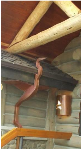
Figure 1 Choose good materials and avoid polluting ones (like this copper downspout).
