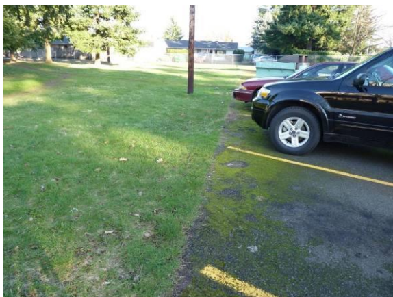
Figure 8 Another accidental vegetated filter strip. The parking lot sheds runoff to the left towards the grassy area. A lack of curbs and additional drainage means all the runoff from the parking lot stays on-site.
