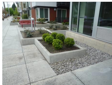
Figure 9 Crushed aggregate can be as aesthetically pleasing as rounded river rock and does a better job at protecting water quality.
