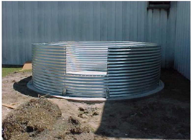
Figure 3 Metal cistern being constructed.
