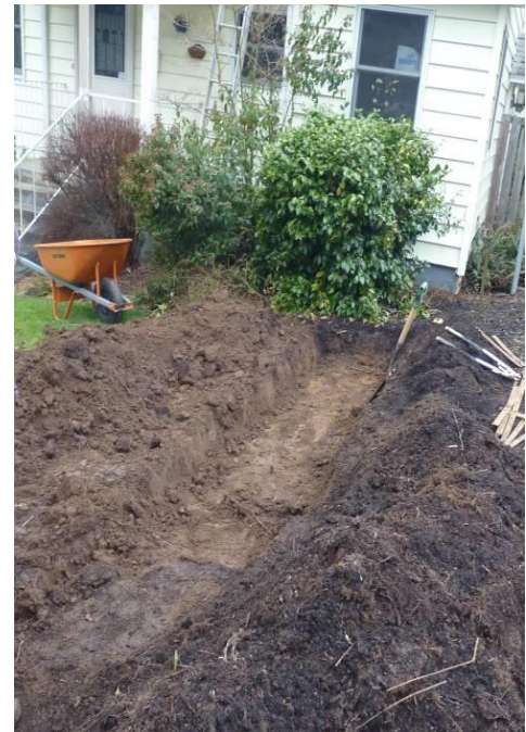
Figure 6. This vegetated conveyance swale will be partially lined, which is why it's so deep.
