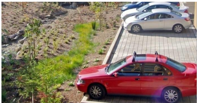
Figure 10 A daylit stream, a rain garden, porous pavement, and native plants all work together to protect water resources on and off site.
