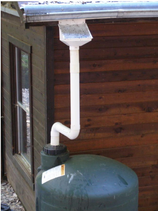
Figure 8 Rain barrel for landscape watering. Note the leaf guard over the gutter screen and strainer basket, which are used to reduce clogging and maintenance.
