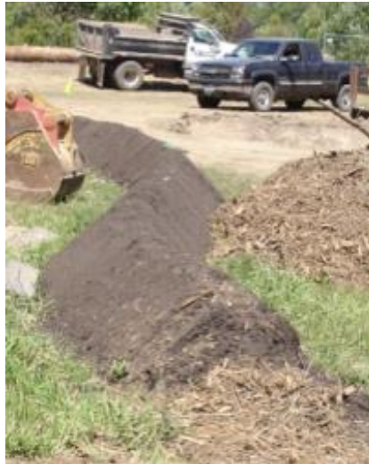
Figure 2 This berm, made of compost instead of ordinary loose soil, is highly effective at reducing sediment transport off-site and can be installed by hand or machine.
