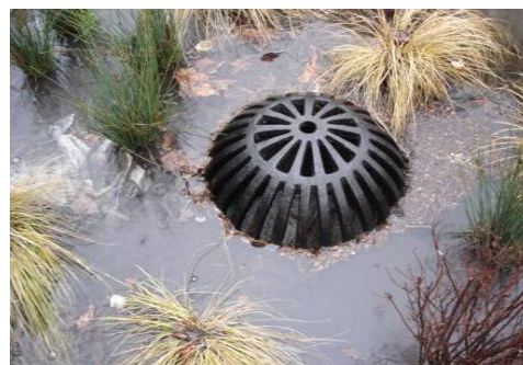
Figure 12 Avoid bark mulch. It floats, carrying pollutants adhered to its surface to downstream waterways.
