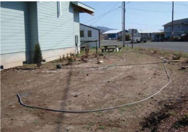
Figure 13 Delineate the rain garden with a hose, strings, stakes, or marking paint. Call 811 to locate utilities.
