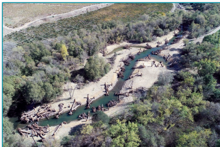
Newly constructed side channel in the upper reaches of Dry Creek which was fully completed in late 2018. Photo Credit: SCWA
