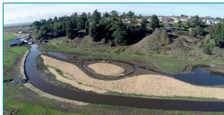
Tide gate replacement, slough channel restoration, and tidal wetland construction in Martin Slough, Eureka, CA.
