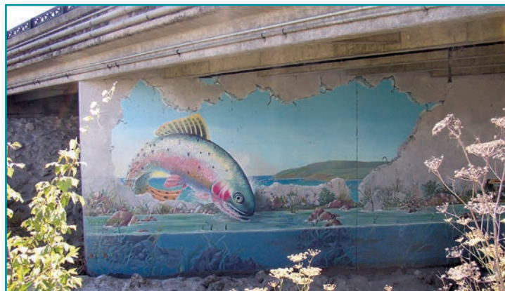
"Breakthrough" mural on Railroad Street bridge over Santa Rosa Creek in the Prince Memorial Greenway. Photo Credit: City of Santa Rosa.
