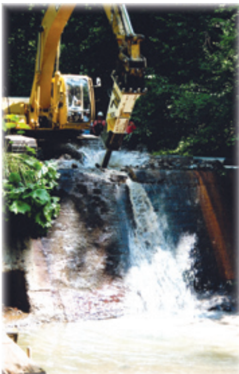
The West Panther Creek Dam on the Mokelumne River is removed as a result of a federal dam relicensing process. Note: SRF does not condone the use of heavy equipment in the riparian zone.
