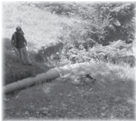
Maintaining & unplugging culverts is an integral part of winter road maintenance.
