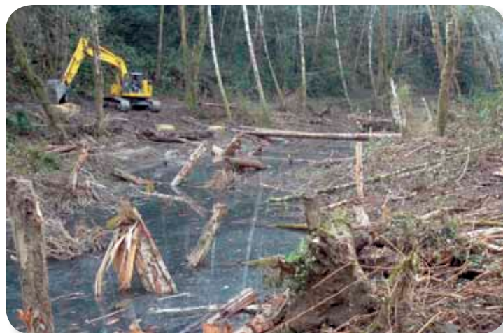
Looking upstream at Rocco Fiori finishing construction of McGarvey Creek Alcove I, a project of the Yurok Tribal Fisheries Program.
