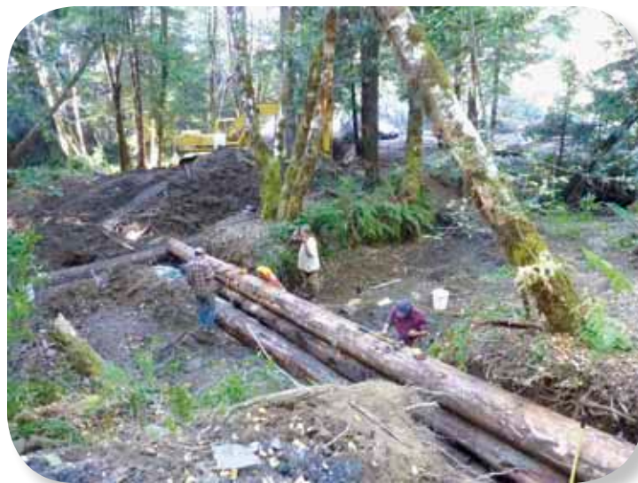
Construction of channel spanning log structure to reconnect floodplain and off-channel habitat in Baker Creek, Mattole River Headwaters.
