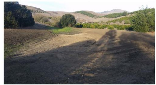
Photograph of a recharge basin under construction on a property adjacent to Santa Rosa Creek. This pilot project was completed in 2015 and is an example of one of the types of successful groundwater recharge projects that would be incorporated in the Middle Santa Rosa Creek Streamflow Enhancement Planning Project.
