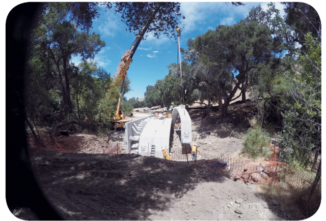
Quiota Creek Crossing 5 ConTech bridge installation on 8/28/18. Photo provided by COMB Fisheries Division staff
