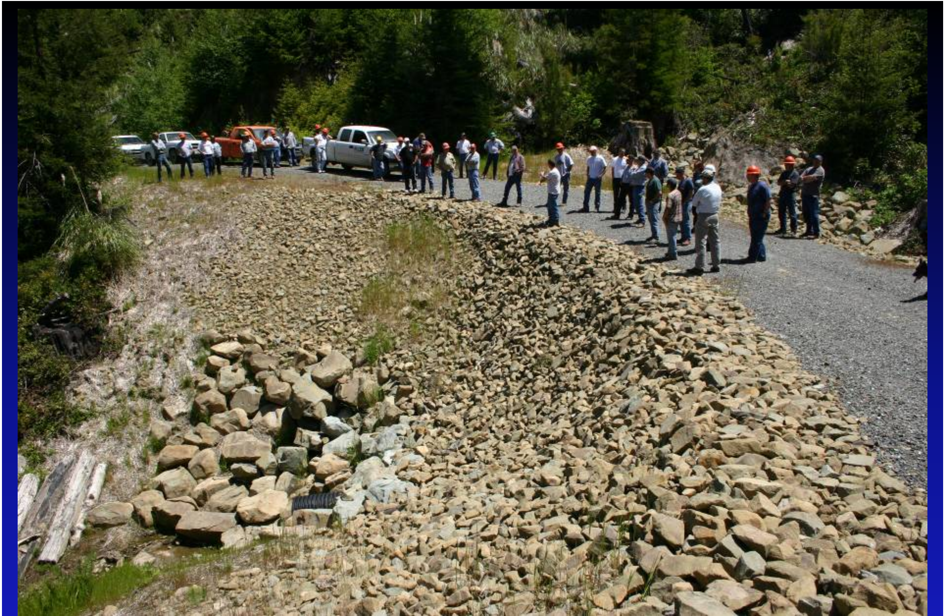
Over-rocked fillslope
