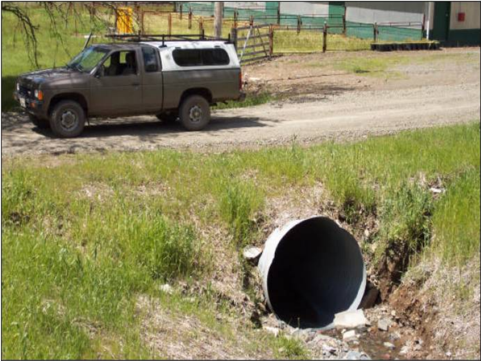
Culvert upgrade: after
