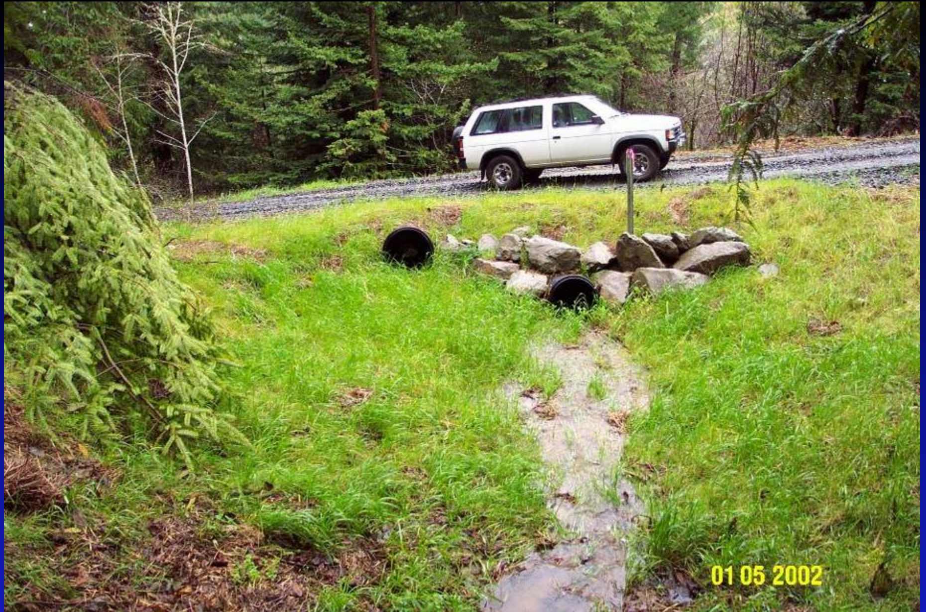
Emergency overflow culvert
