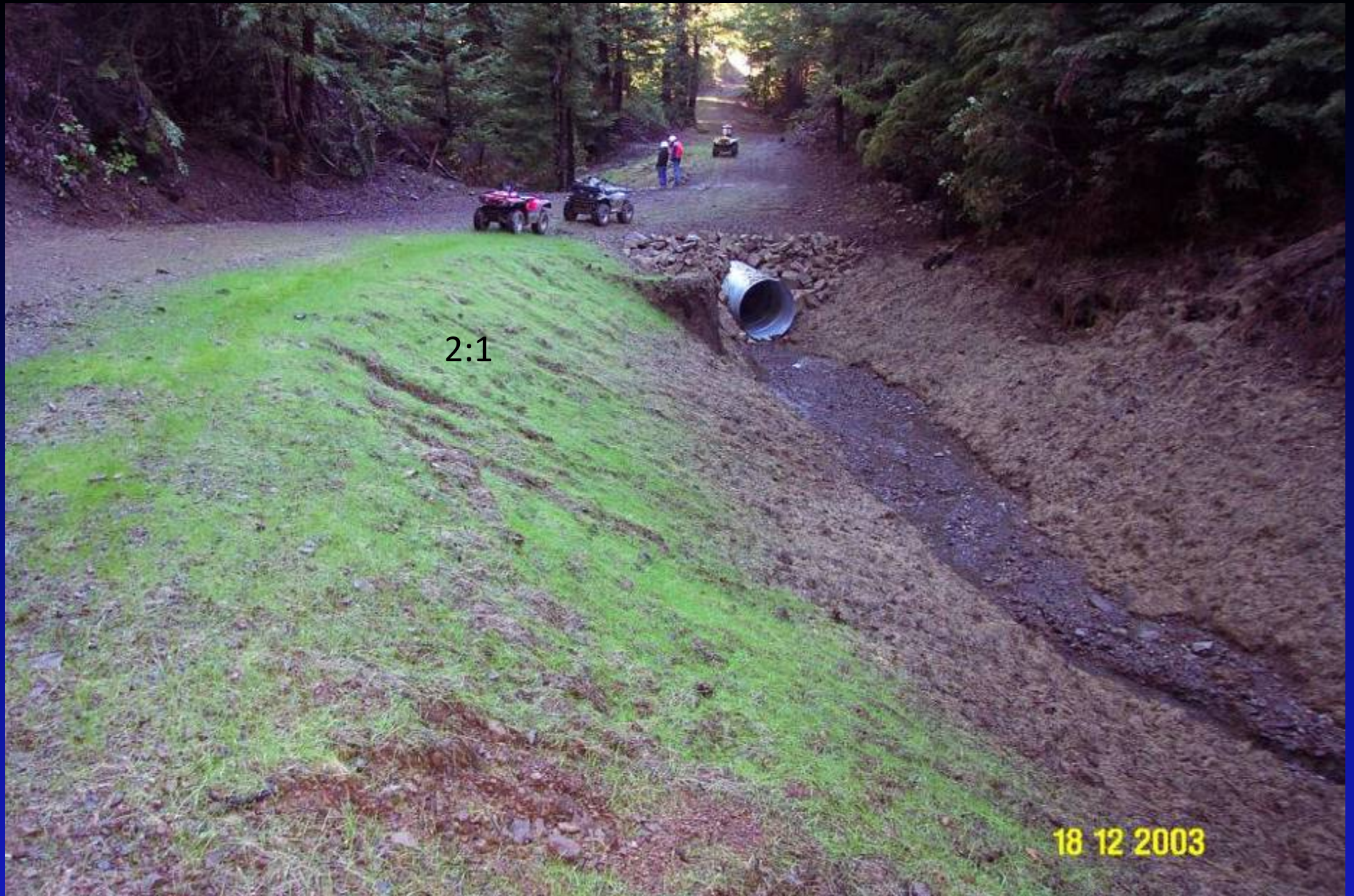
Upgraded stream crossing
