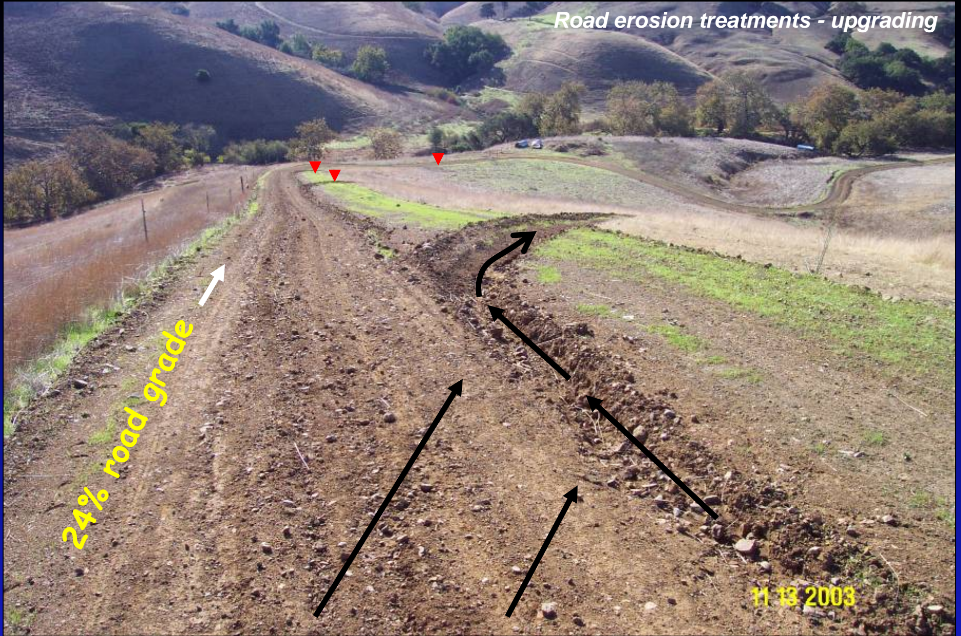
Berm breaks on a fall-line road
