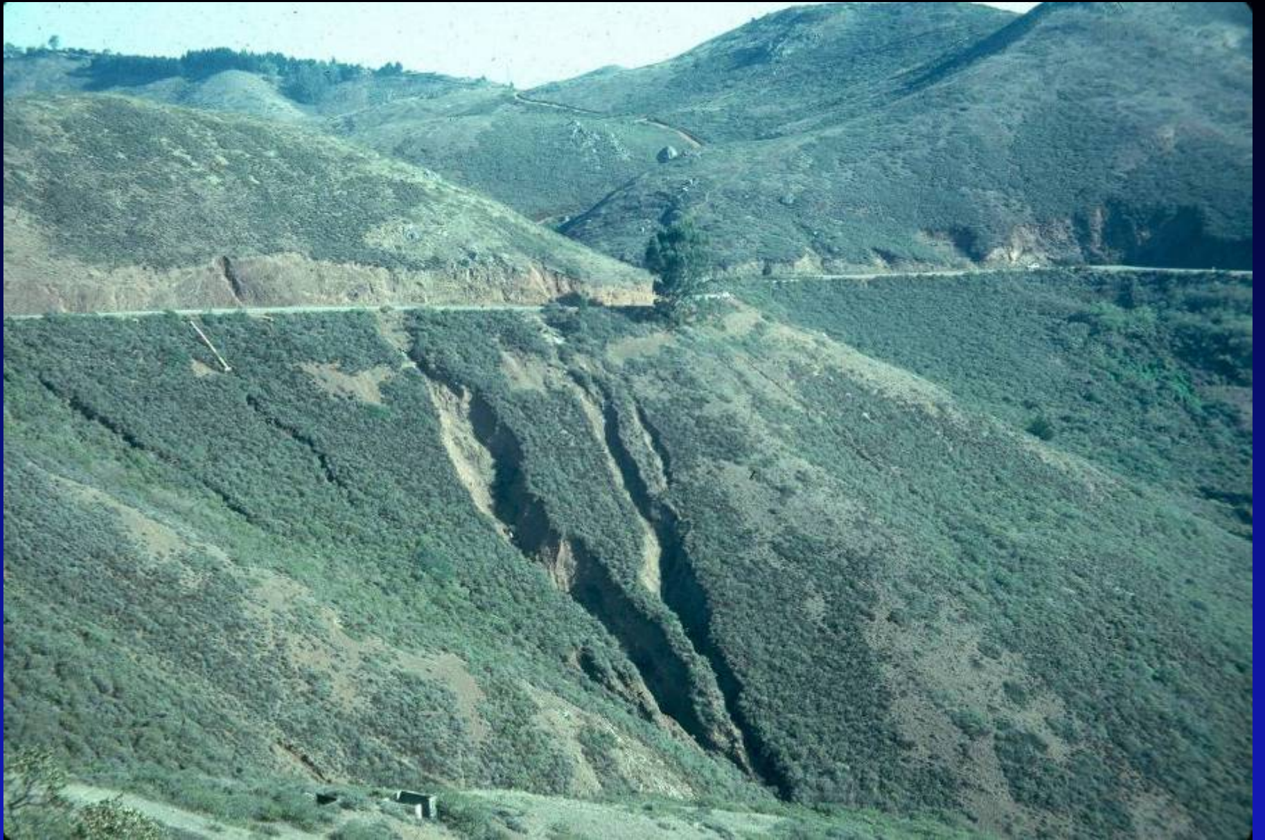
Gullies from road surface runoff
