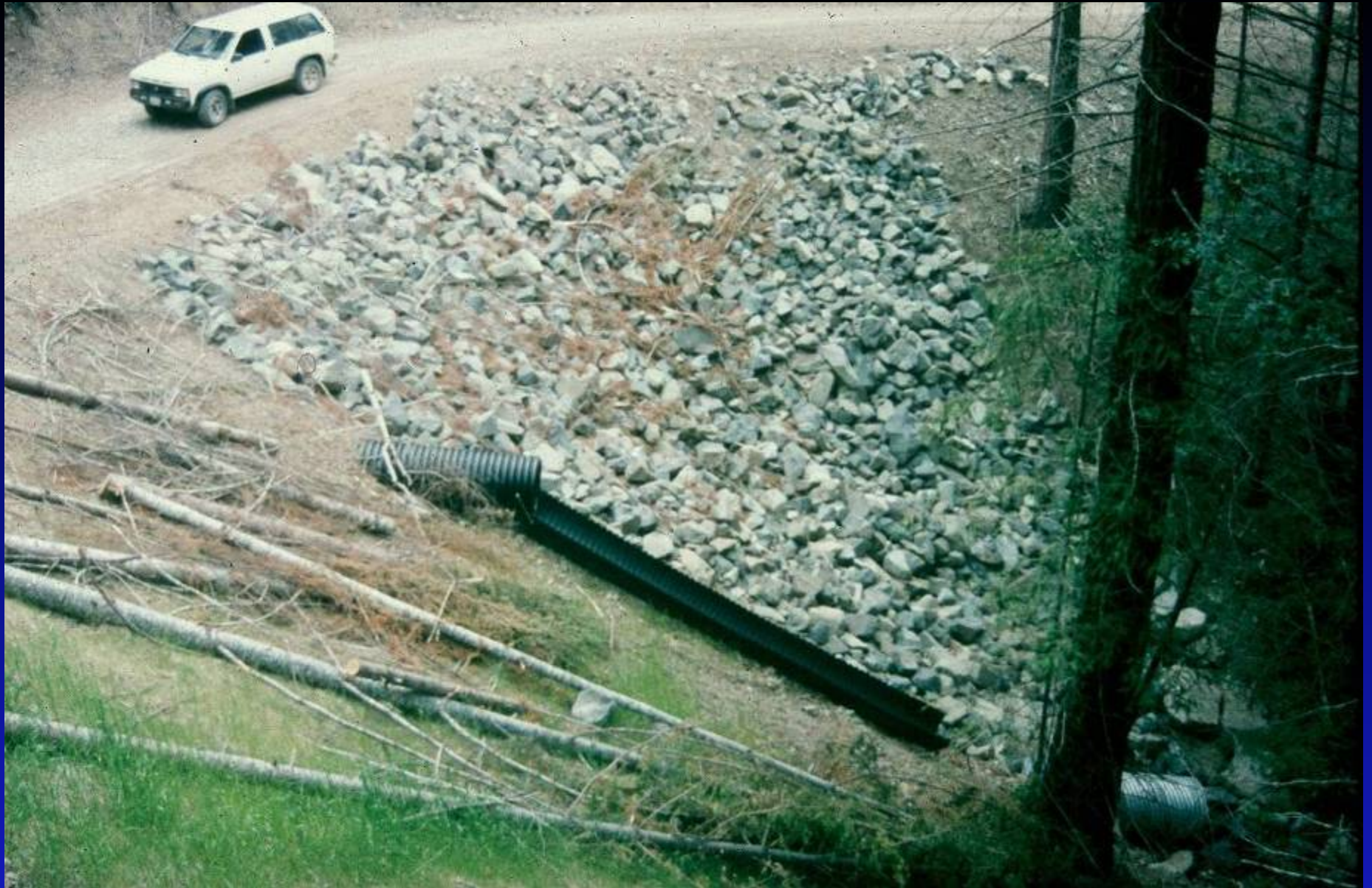
Emergency overflow culvert
