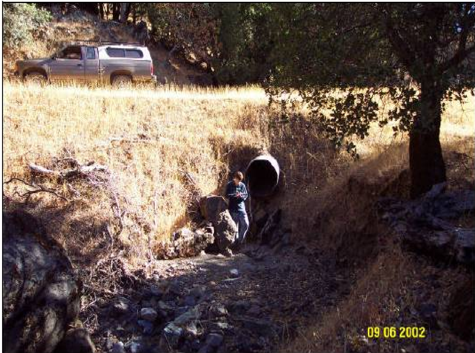
Culvert upgrade: before
