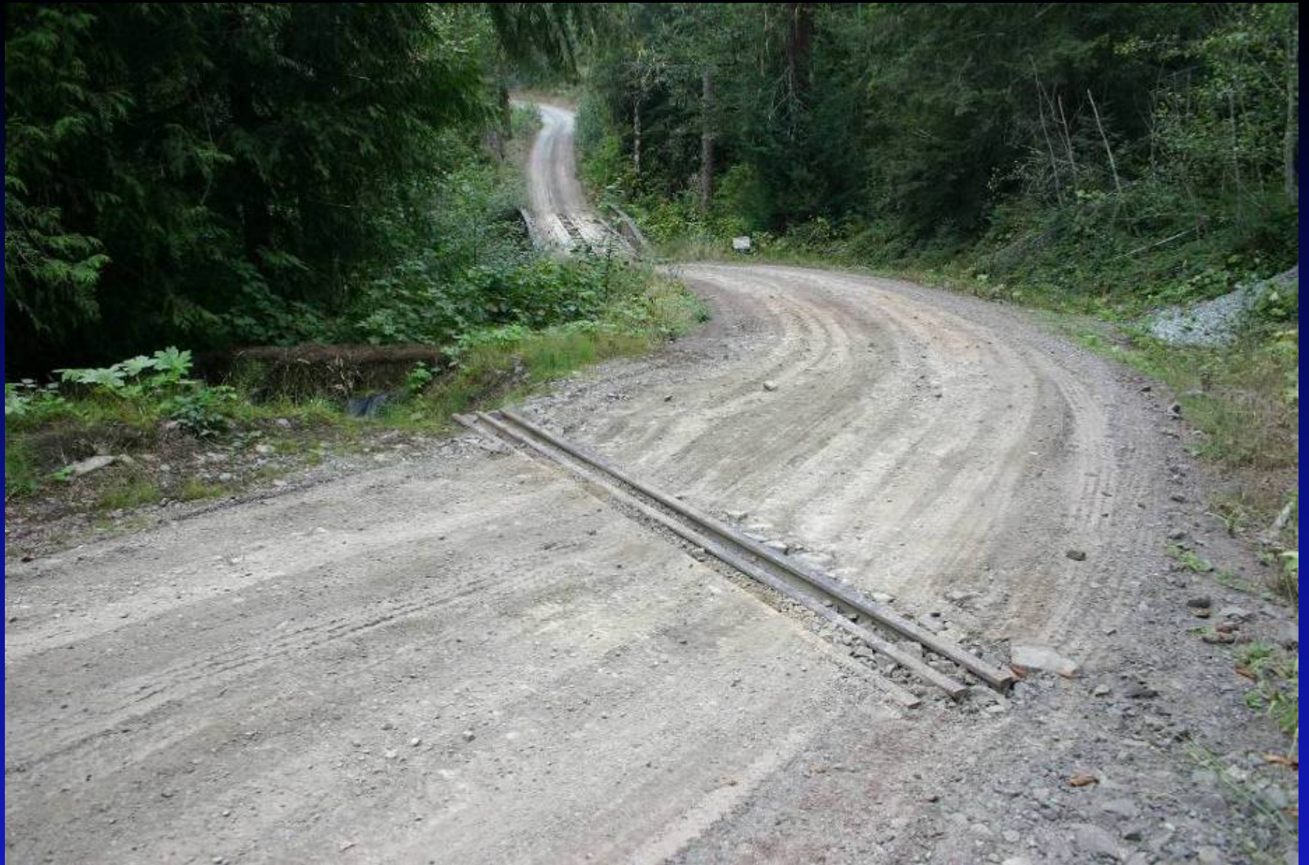
Slotted road drain
