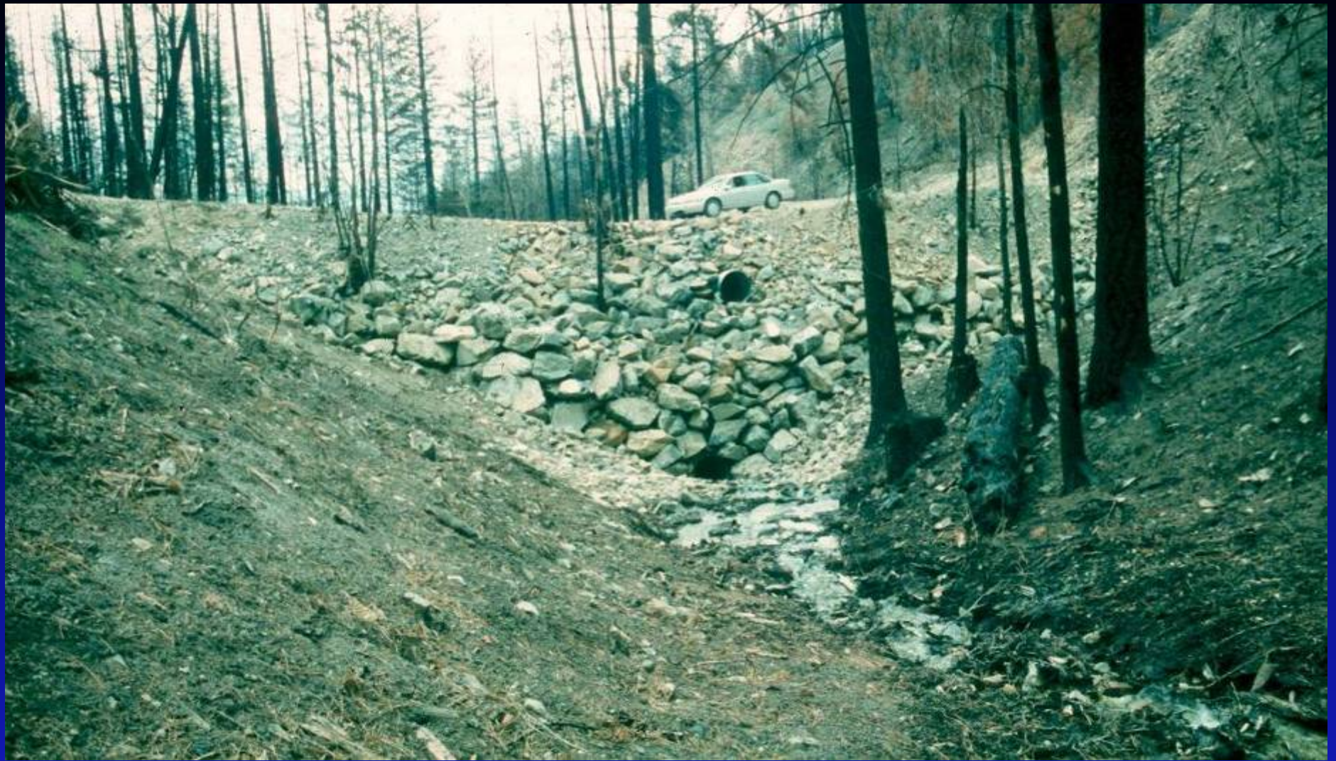
Emergency overflow culvert
