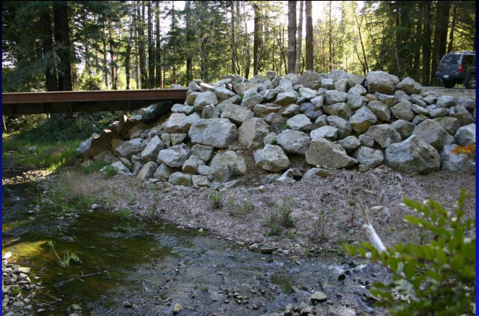
Armoring bridge abutments
