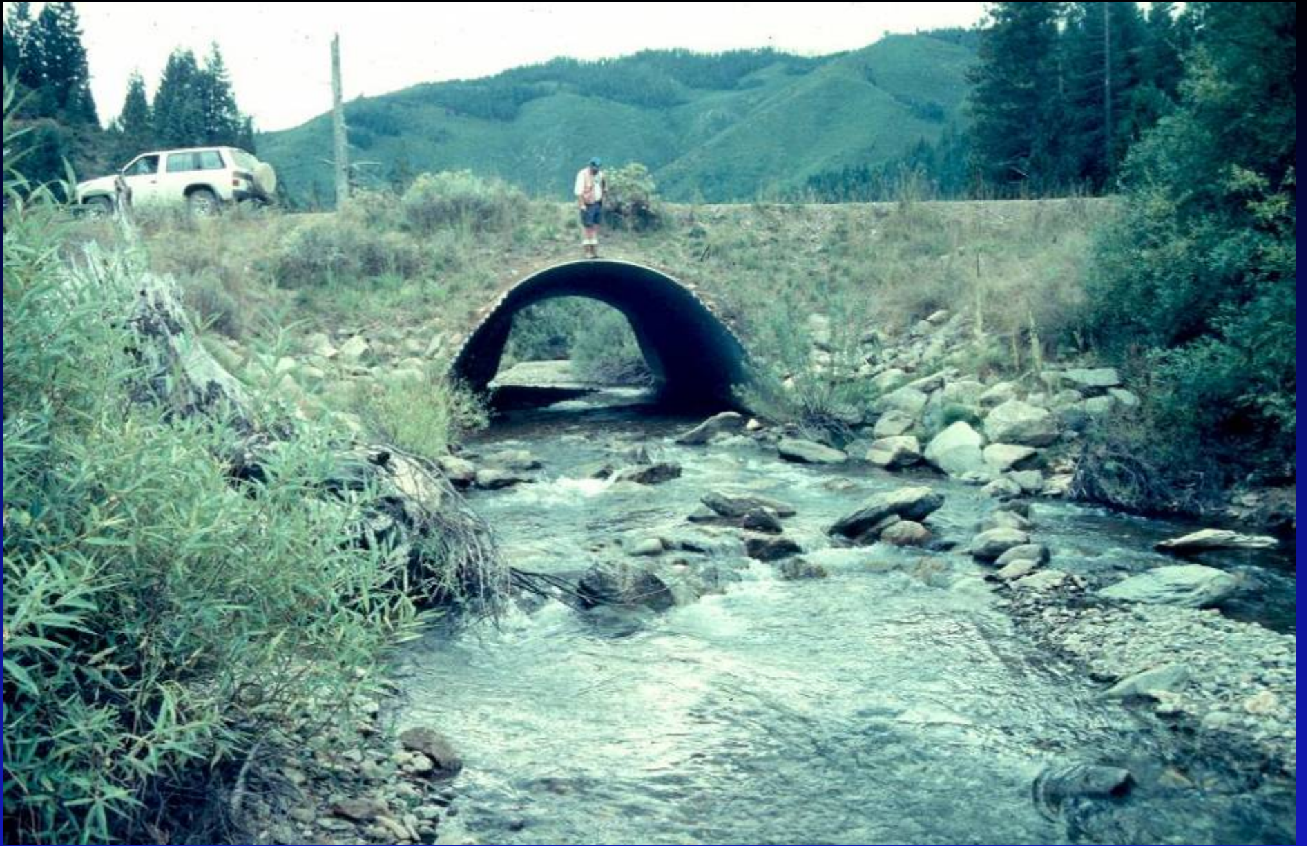
Plate arch (bottomless arch)
