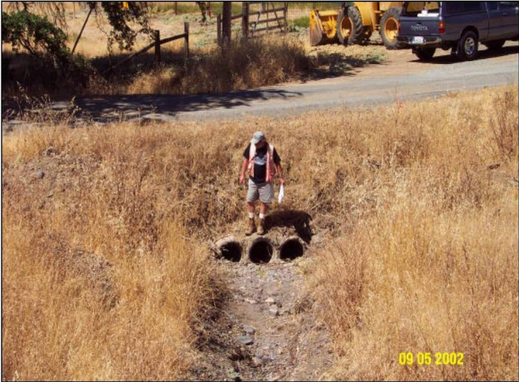
Culvert upgrade: before
