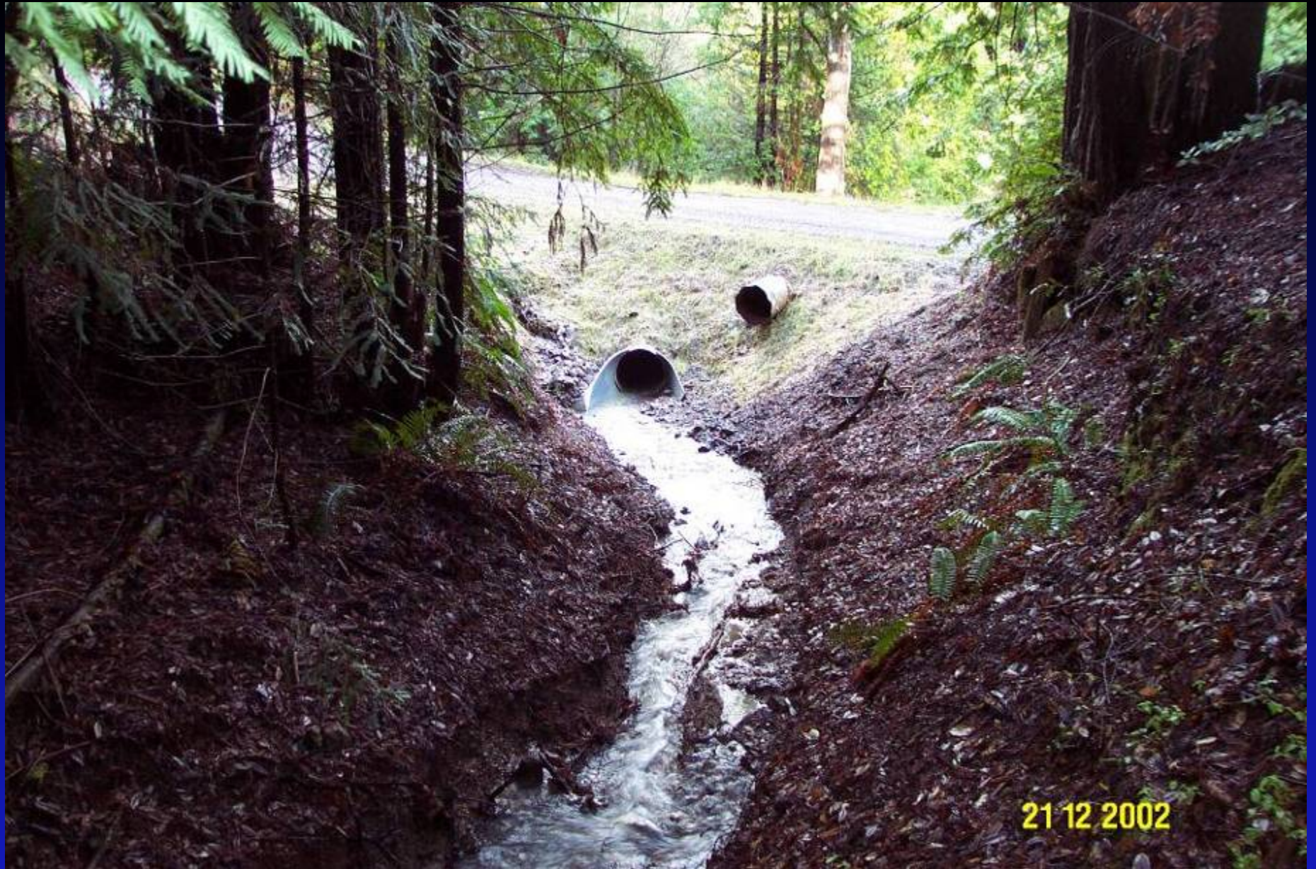
Emergency overflow culvert
