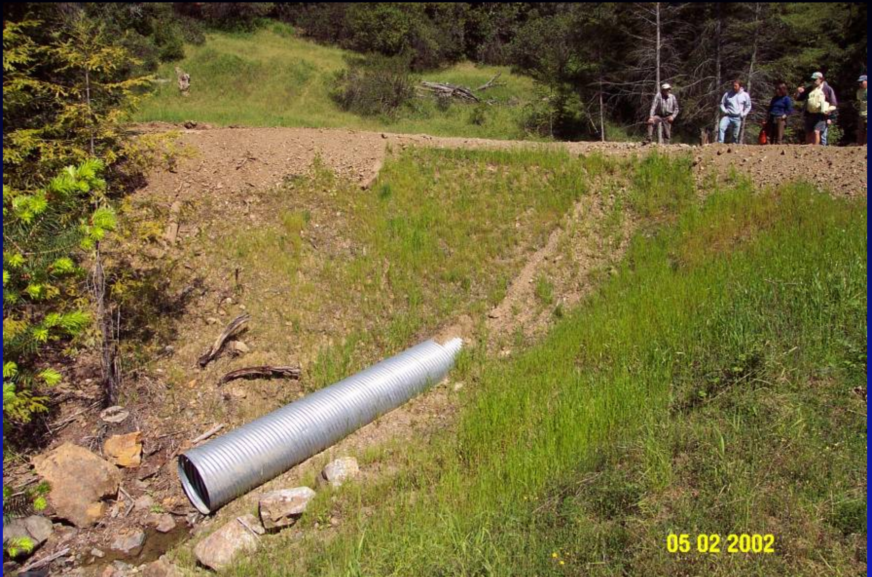
Culvert extension and fillslope grade
