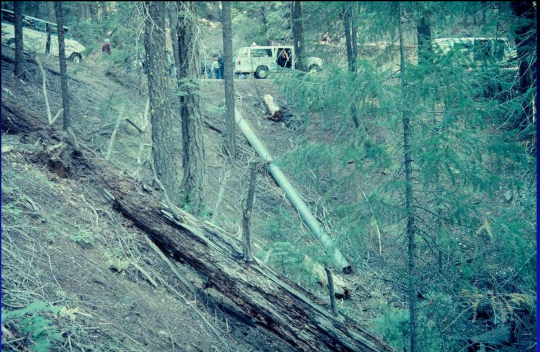
Shallow culvert with downspout
