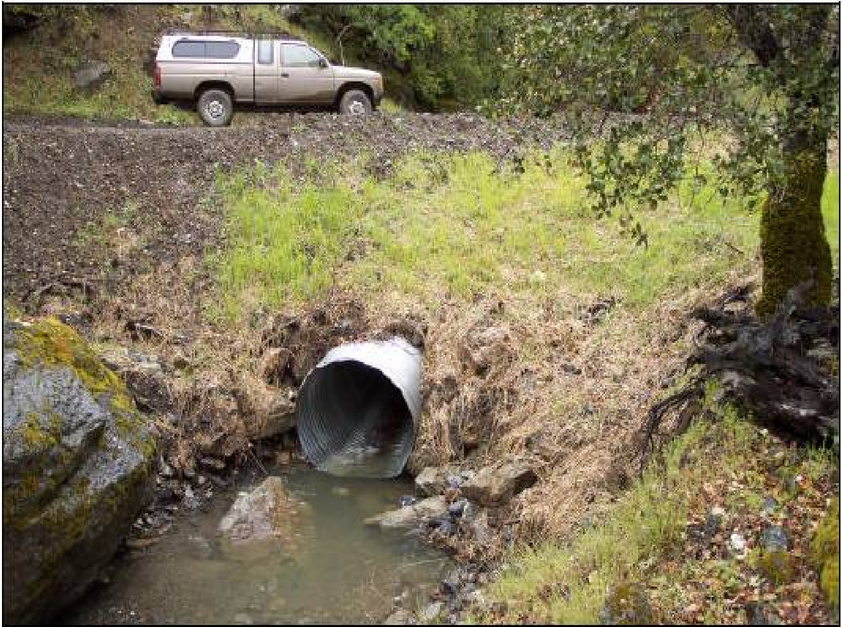
Culvert upgrade: after
