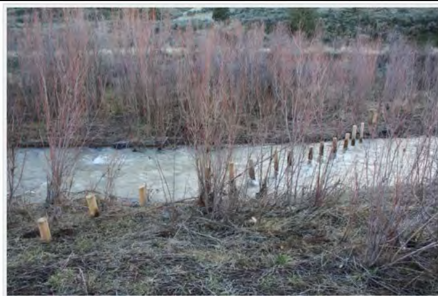
Incised Channel Restoration, Bridge Creek, Oregon (Source: Pollack et al., 2012)
