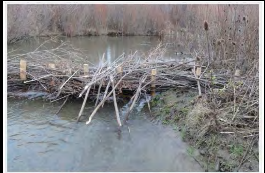
Debris Retention Device by Knuass, Bavarian Alps (Source: Wallerstein, Thorne and Abt, 1996)
