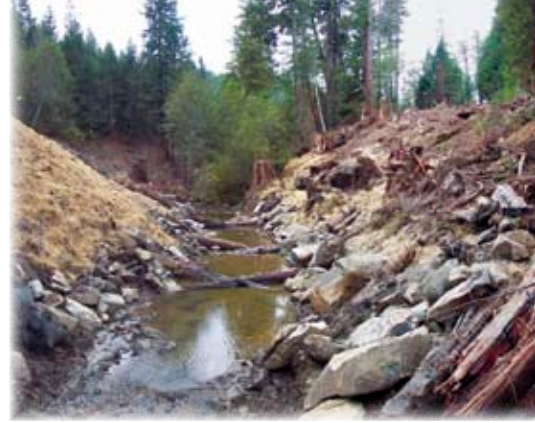
A Pacific Watershed Associates' erosion control project.
