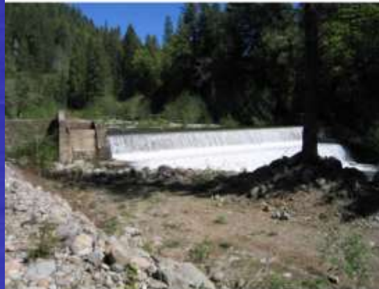
Figure A7.1-5. Hendricks Diversion Dam.
