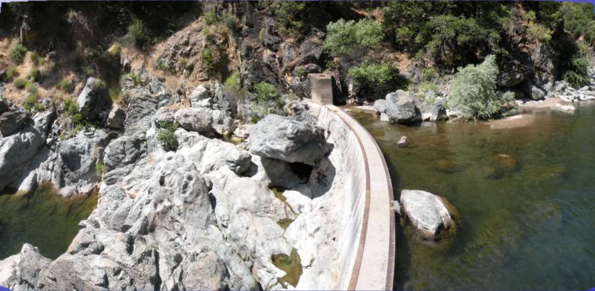
Centerville Head Dam 1150 feet elevation
