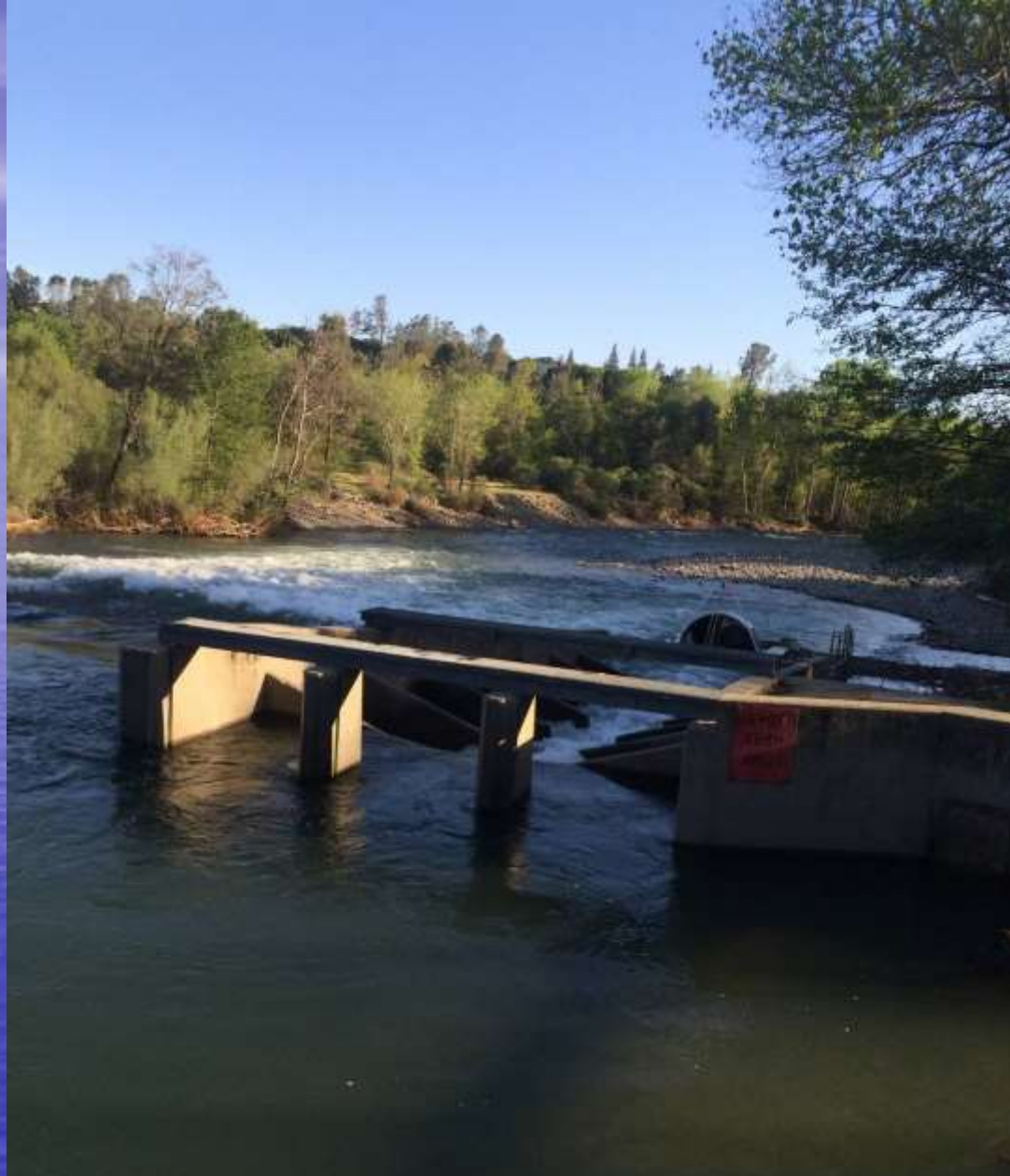
Fish Ladder/Irrigation Diversion
