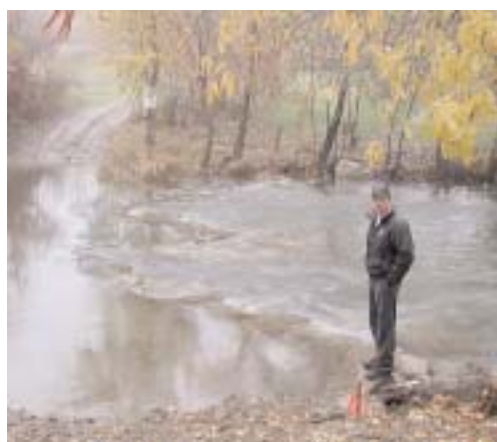
The weir at Hasbrook Crossing is one of the sites that will be visited during the Putah Creek tour.
