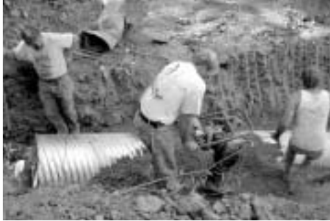
Restorationist Bill Eastwood overseeing a culvert replacement.
