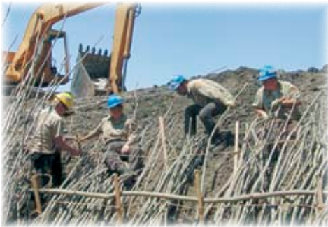
Participants will visit bioengineering projects completed by the California Conservation Corps and will have the opportunity to construct willow walls.
